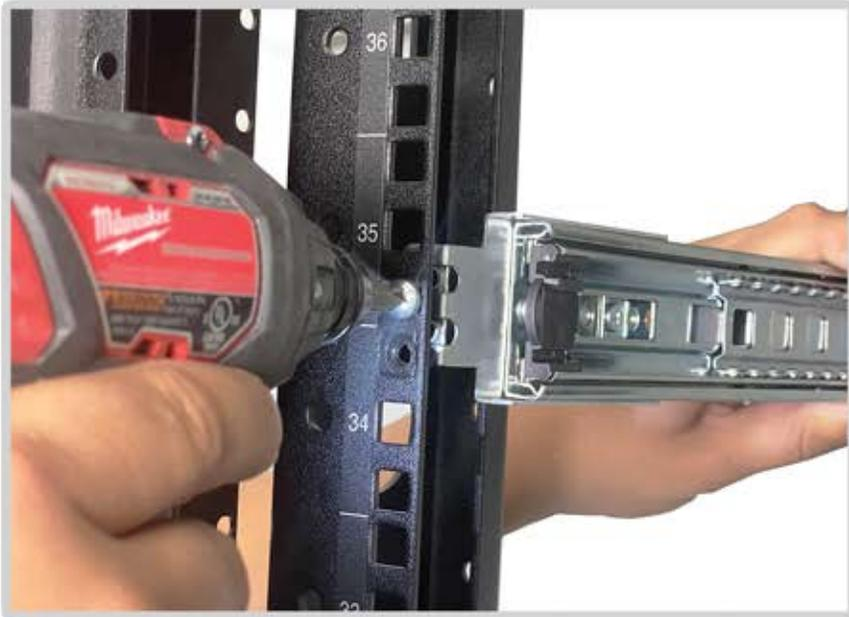
Place 1x 10-32 x 1/4 screw onto the bit of your screw driver, press it into the top hole of the Front Offset Clip (you may have to spin the screw to get it to thread into the clip) and then hold the rack slide assembly in position, and loosely install the first 10-32 screw.
